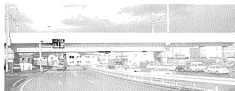
[JR環状通り架道橋]
